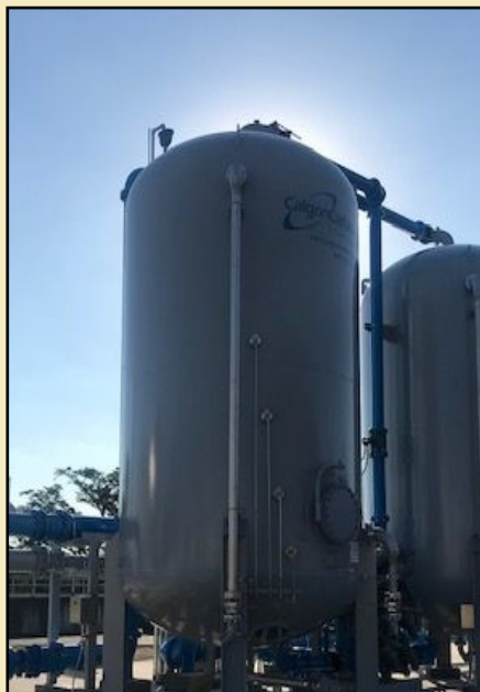
Granular Activated Carbon Filtration System
