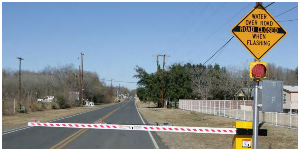
Figure 63. Flood Detection System Automated Gate Example
