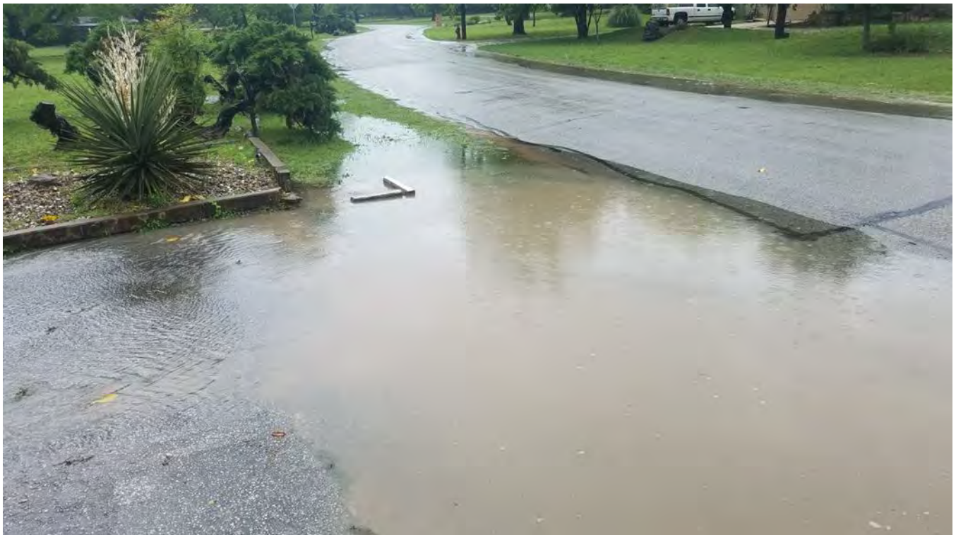
Figure 58 - Inadequate Inlet Capacity at Jack Drive - April 24, 2019 (Source - Residents)
