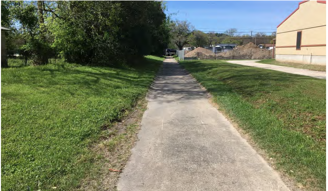
Figure 51 – Undersized Concrete Ditch at Lois Street
