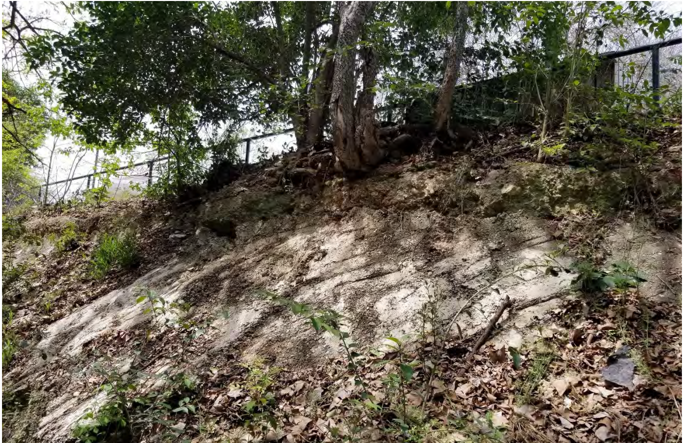
Figure 48 – Unstable Side Slope for Take It Easy Channel
