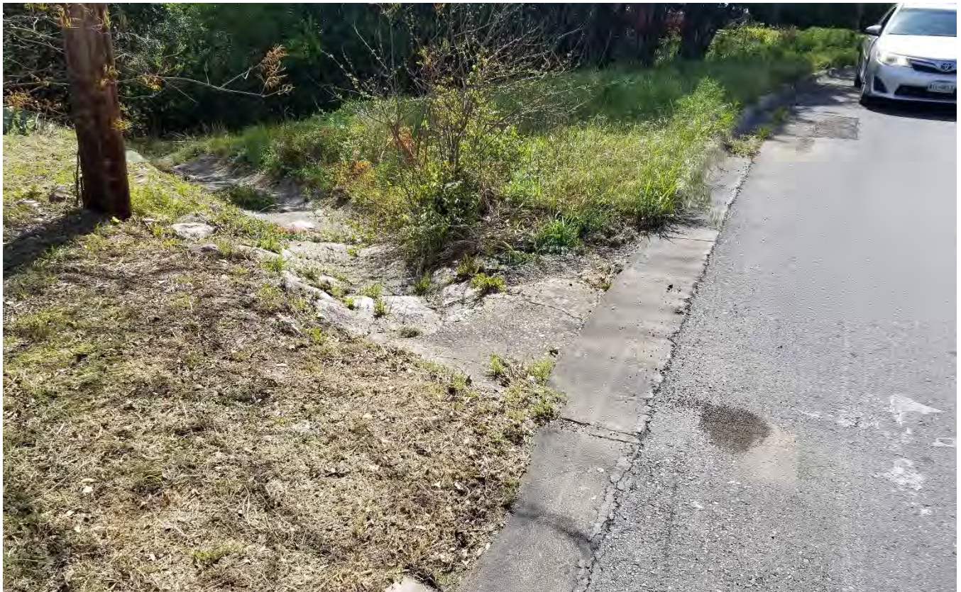
Figure 55 – Circle Avenue Earthen Channel Erosion
