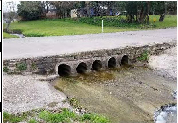
Existing 5 - 24" RCP Culvert (Facing U/S)
