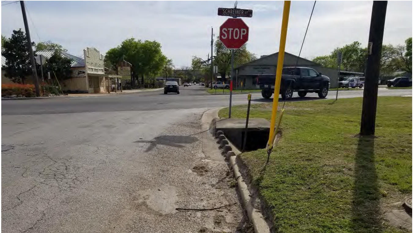
Figure 42 – Stormwater Inlet at Clay Street
