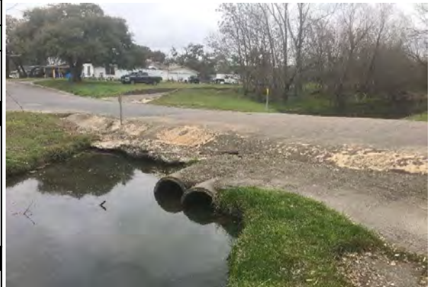
Existing 2 - 24" RCP Culvert (Facing D/S)
