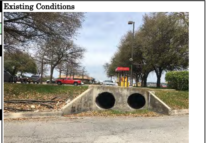
Existing 2 - 36" CMP Culvert (Facing D/S)
