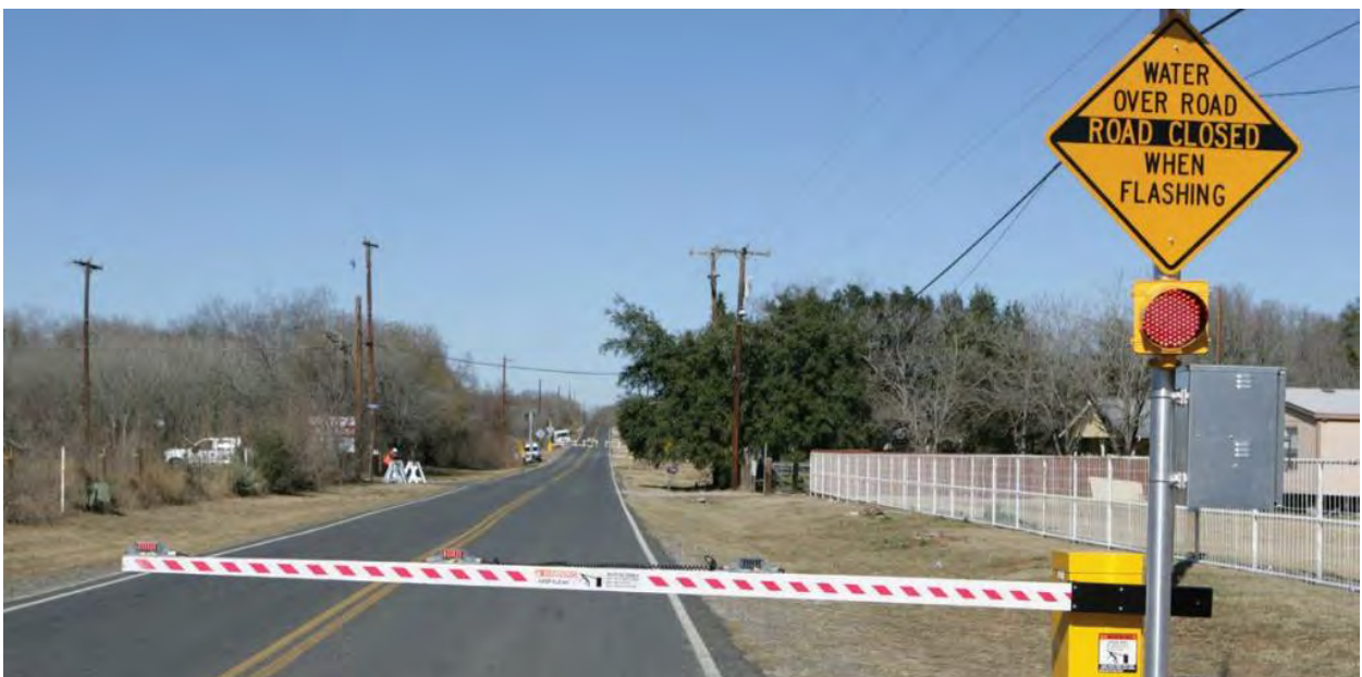
Figure 65 - Flood Detection System Automated Gate Example
