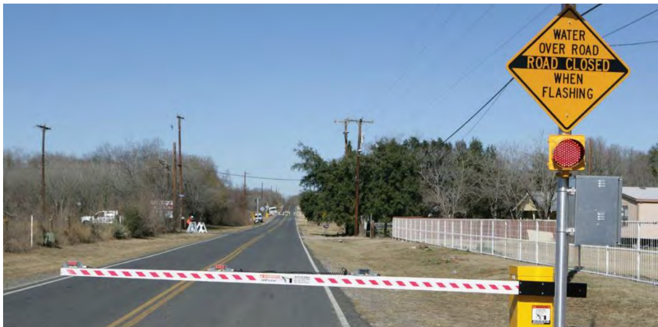
Figure 64 - Flood Detection System Automated Gate Example
