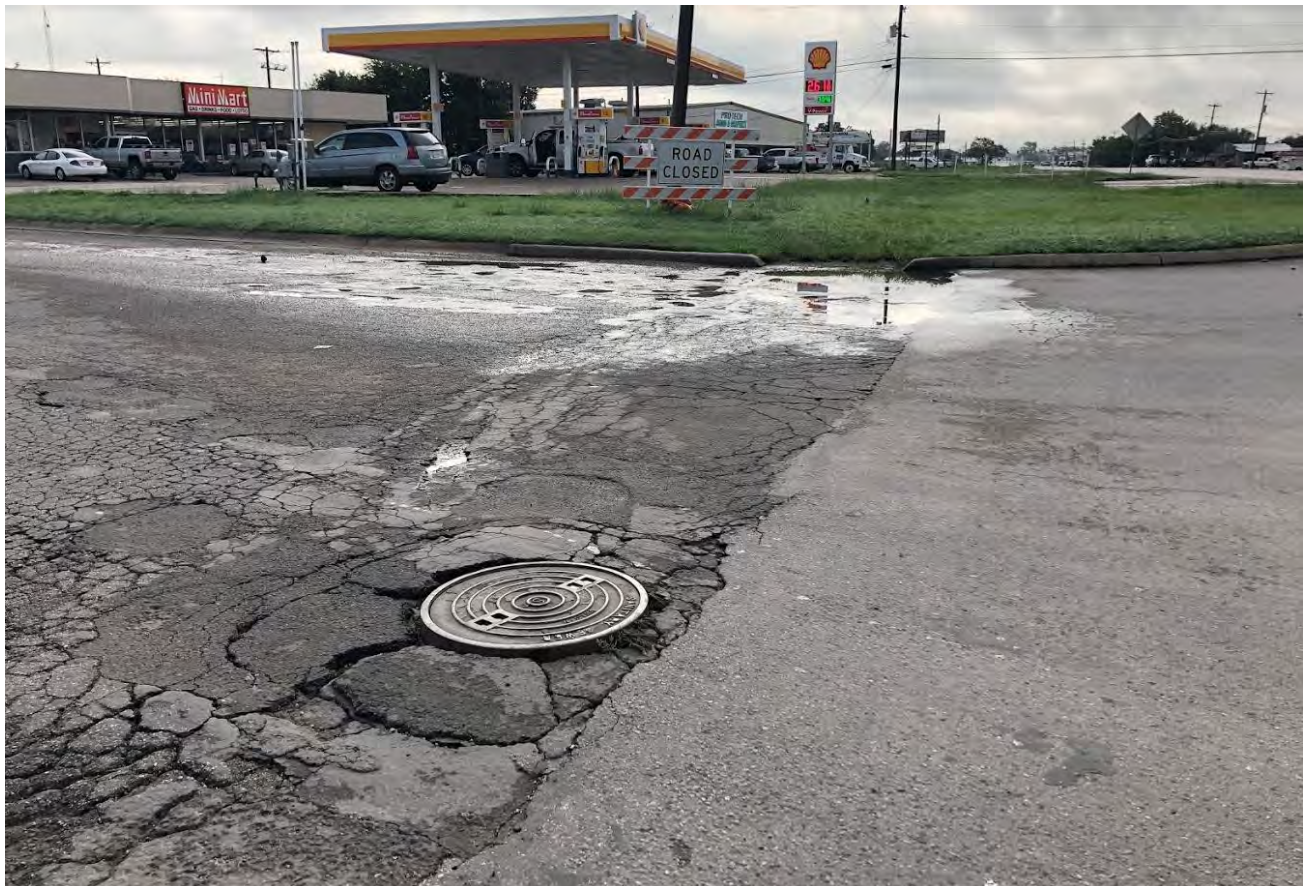
Figure 61 – Ponding at Coronado Drive at Junction Highway Intersection (Facing Southeast)
