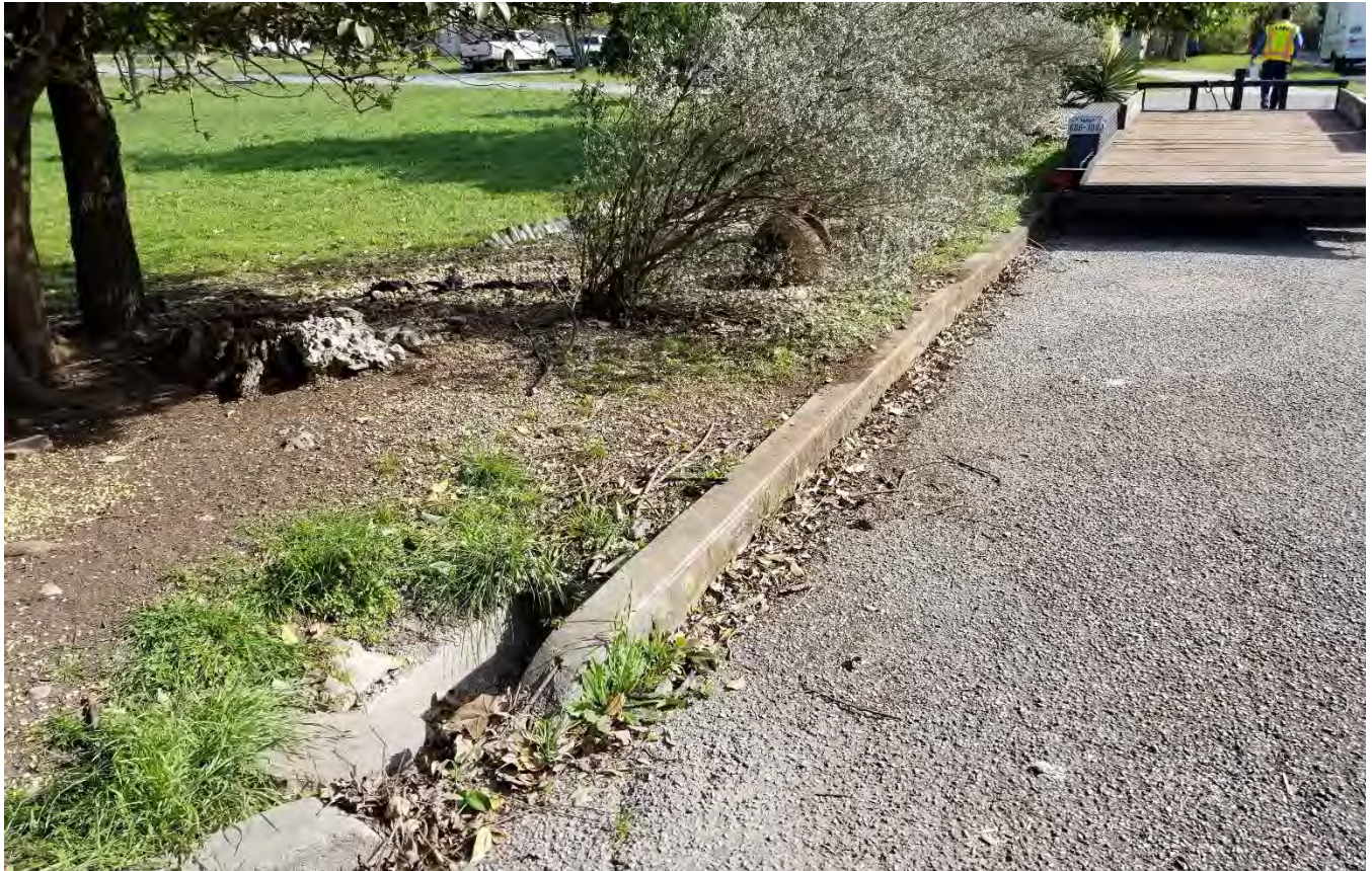
Figure 57 – Outflow of Undersized Storm Drain at Jack Drive Facing Upstream
