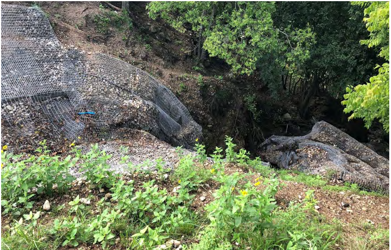
Figure 37 – Channel Failure at Guadalupe River Bank
