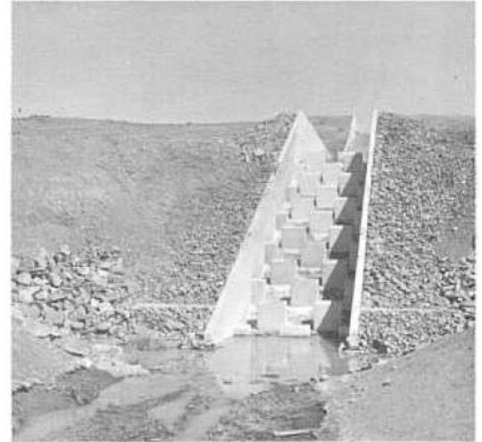
Figure 66 - Baffled Chute Energy Dissipater (Source: USBR EM-25)
