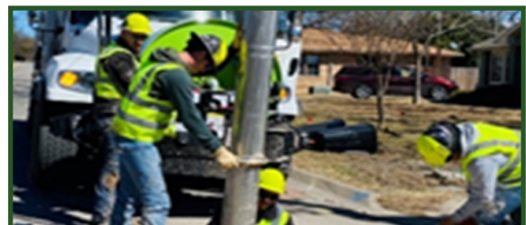
Wastewater Collections performing a Hydro Excavation to repair a customer's service line.
