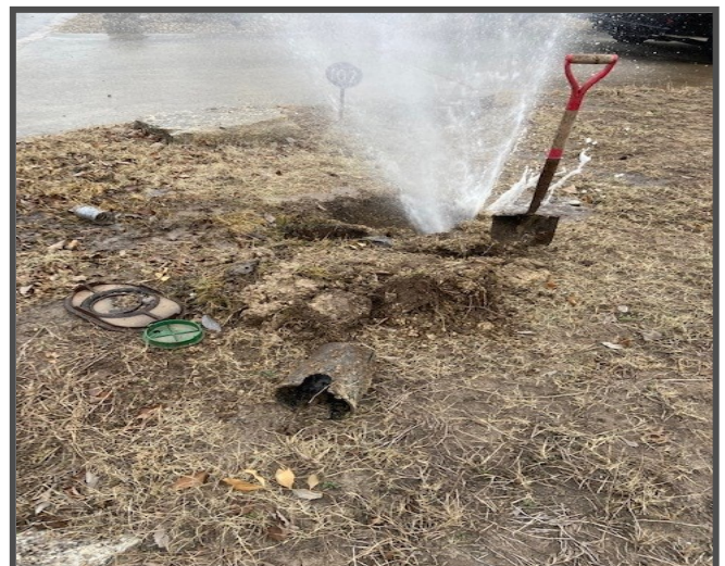
Utility Billing Meter Technicians responded to a busted curb stop.
