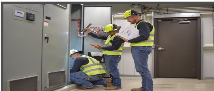
Operators are performing voltage checks to ensure that pumps are within operating parameters.
