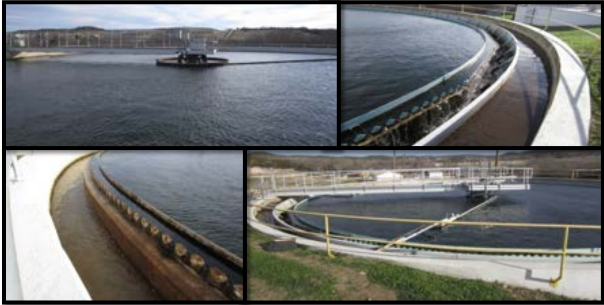
Figure 6.5 Clarifier No. 1 (right) and Clarifier No. 3 (left)
