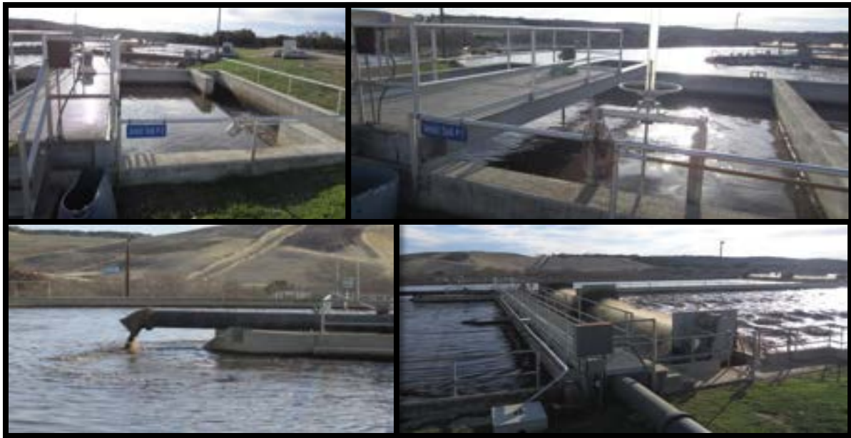
Figure 6.4 Anoxic Tank (top) and Oxidation Ditch (bottom)
