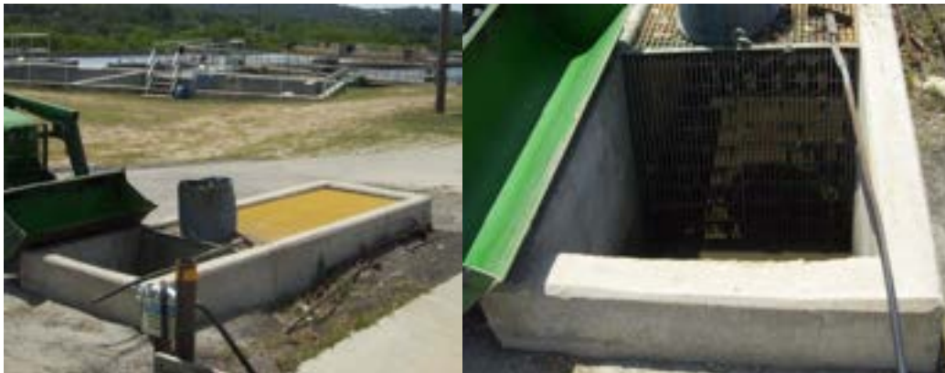
Figure 7.3 Existing Septic Screening Structure
