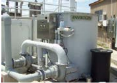
Figure 7.2 Existing Odor Control Device
