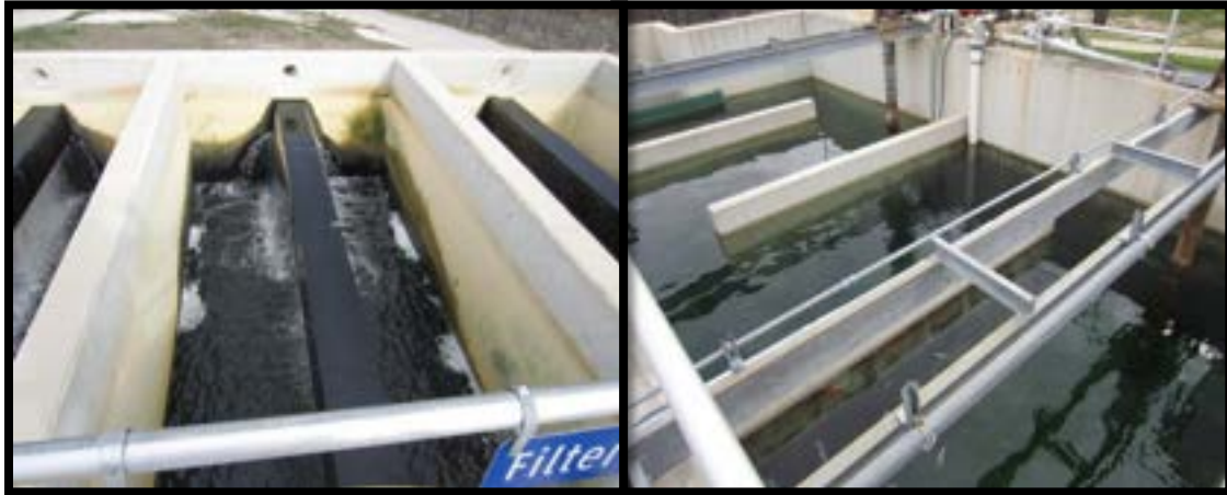
Figure 6.6 Effluent Filters (left) and Chlorine Contact Basin (right)
